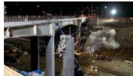
Video: Carmageddon bridge demolition
