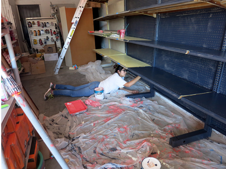
Transforming the interior of Euclid Market.
